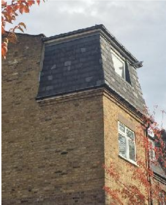
8 Holmdale Road - Back Dormer
