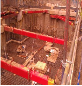
1-6 Clay Street, London 4m deep basement construction
