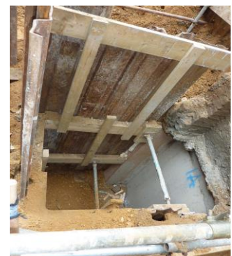
1 Southwick Yard W2 Underpinning/retaining walls - new residential lower ground floor
