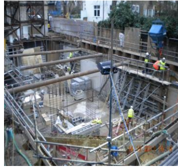
60 Addison Road, Holland Park 4m basement with façade retention
