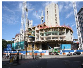
Westminster Park Plaza, London Construction of new luxury hotel by top-down method incorporating 4 basement levels
