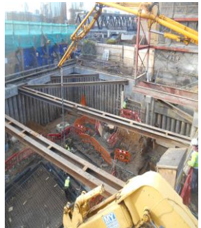
58-66 Cheshire Street, London 5m deep basement construction next to railway line
