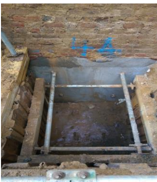
1 Southwick Yard W2 Underpinning/retaining walls - new residential lower ground floor
