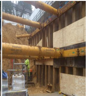
12 The Grove, Highgate 6m deep basement construction
