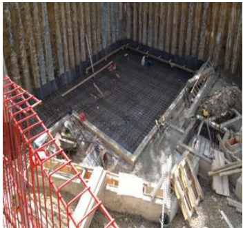
1 St Kildas Road N16 New single basement office facility
