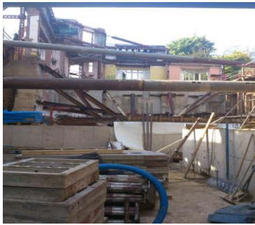
15 The Bishops Avenue 4m basement with façade retention
