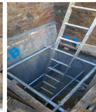
1 Southwick Yard W2 Underpinning/retaining walls - new residential lower ground floor
