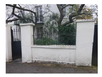
3.2 At the junction of the boundary pier and plinth wall to No 47, there is a wider vertical crack, Category 3, medium, which does require repair.
