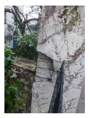
3.5 The frontage plinth all has face brickwork to the rear, garden, face. The pointing is in very poor condition, eroded, loose and missing and requires repointing to the entire length.
