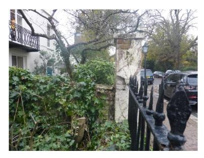
This clearly grew against the wall 'pushing' it over as it grew. A 2m length of the wall now has a significant bulge and is leaning approximately 100m from the vertical.
