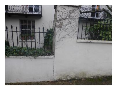
3.3 Coincident with a vertical crack to the front plinth wall, lefthand side of the pedestrian gate, is a crack in the coping. There is a small cherry tree to the front garden, close to the wall. Given the crack pattern present and undulating ground paving this is likely to be the result of tree root damage. However the cracks currently are minor although the wall is neither plumb or level.
