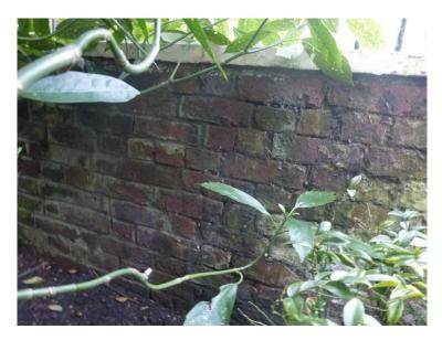
3.6 The most significant damage is to the front garden separating wall. A prior existing holly tree has been removed although part of the trunk remains.
