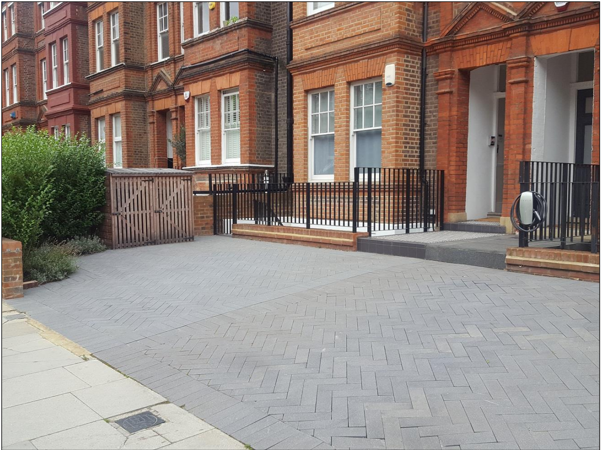
Photograph 7: 63 Goldhurst Terrace frontage.
