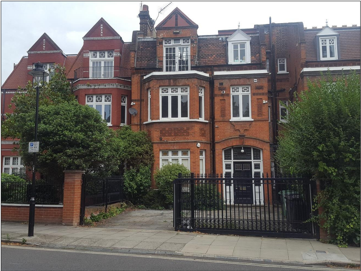
Photograph 2: The frontage of the Appeal Site (looking north).
