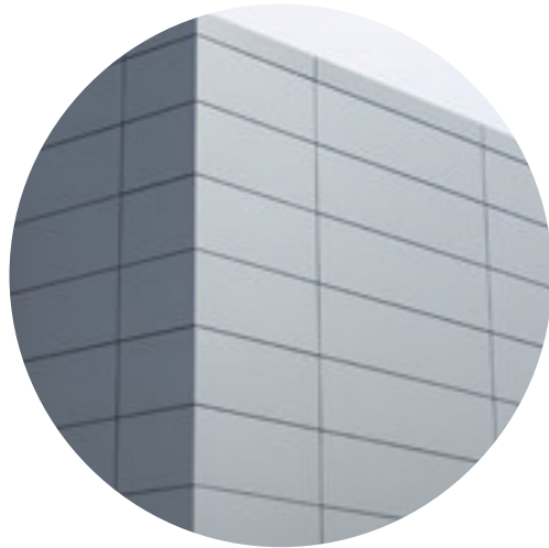
PLANT ENCLOSURE ( SIDE & REAR ELEVATIONS ) POLYESTER POWDER COATED ACOUSTIC PANELS - GREY
