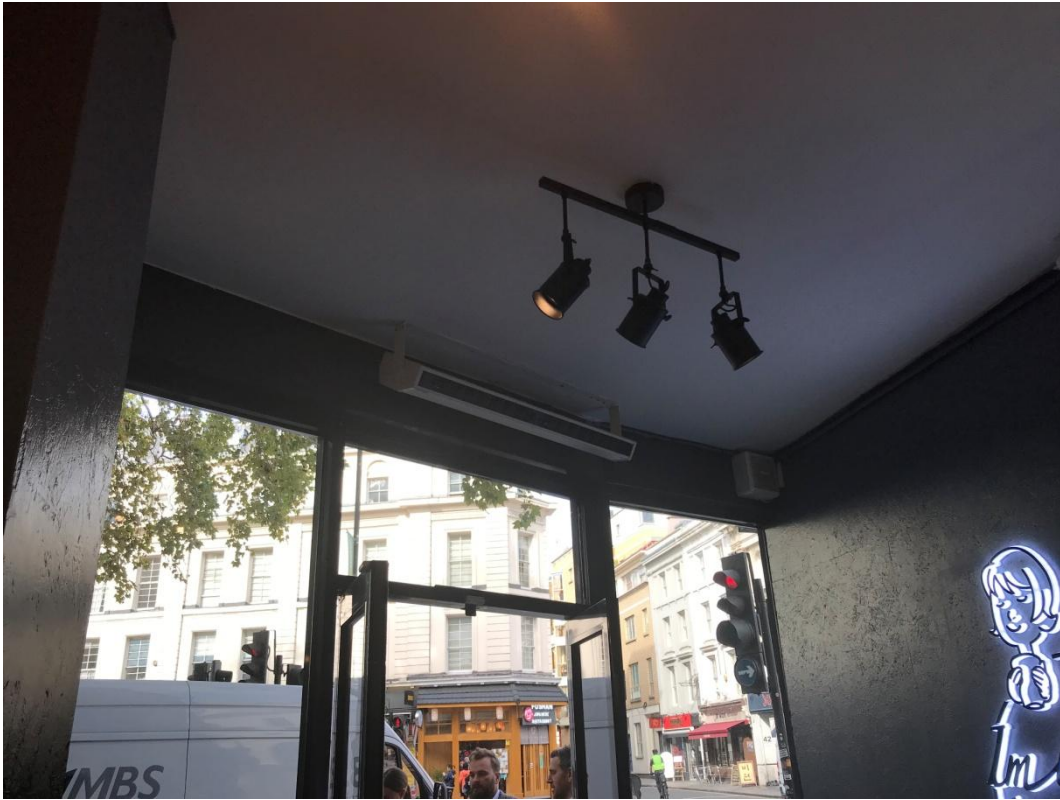
Fig 10 The AC cassette and extractor fan at high level behind the shopfront.
