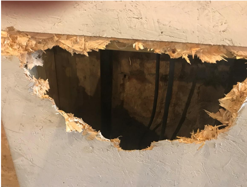
Fig 5 Modern sterling board boxing around existing pipework and cabling.
