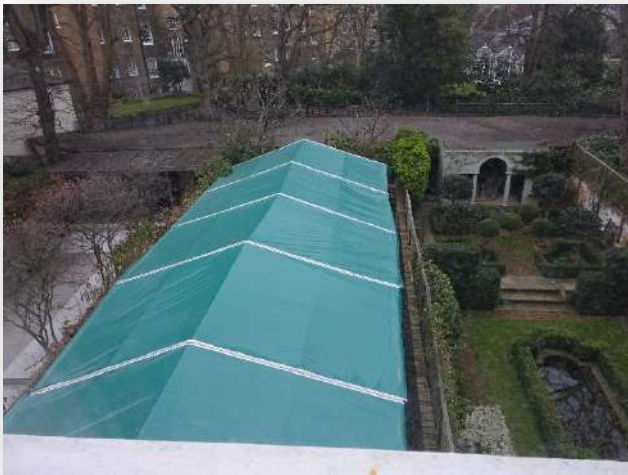
Temporary Cover to Works Area
