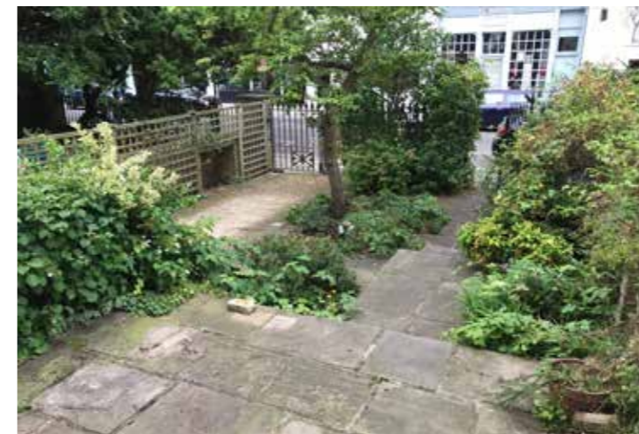
No. 178 Existing front entrance
