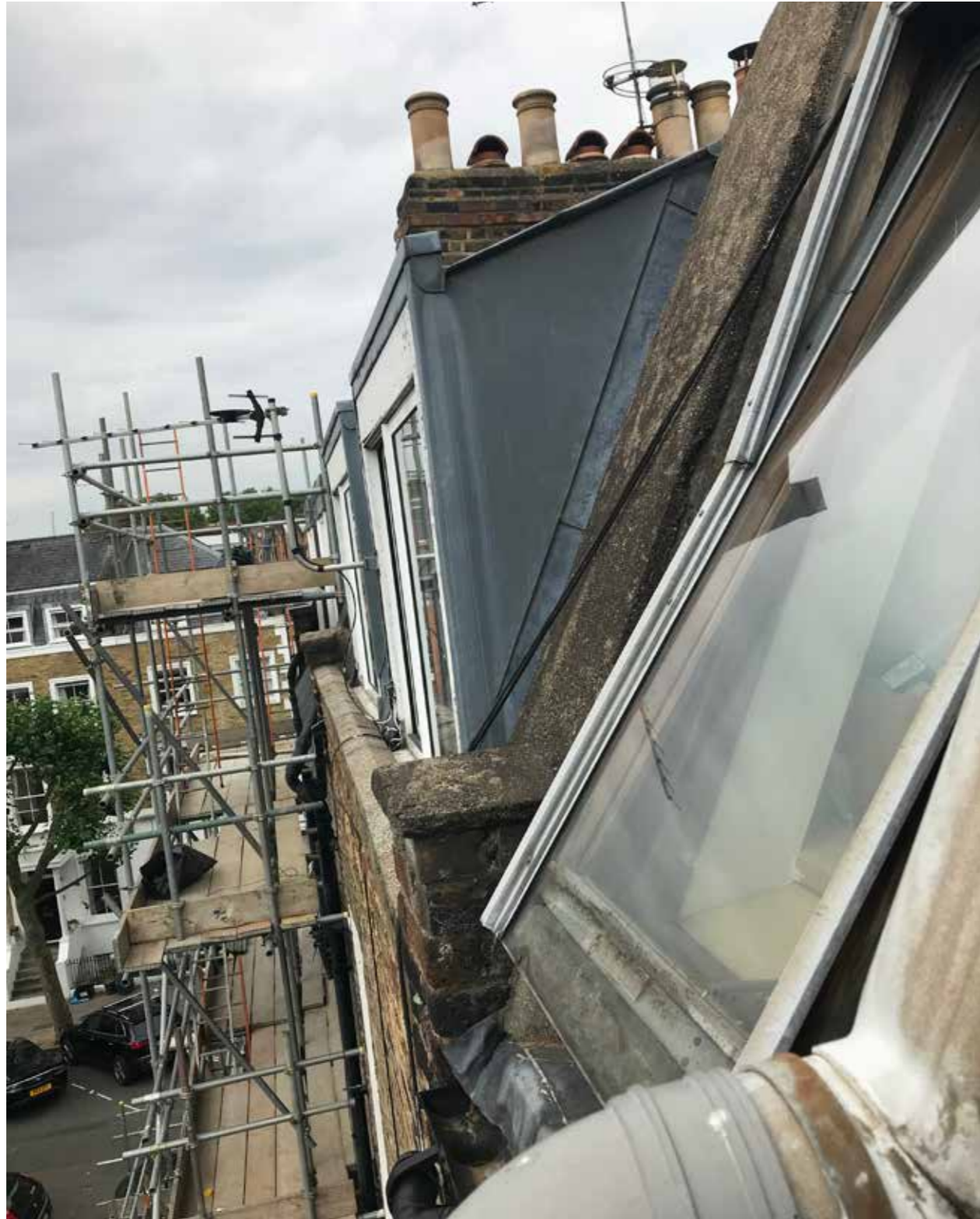
No. 176 Existing mansard roof with dormer window extension
