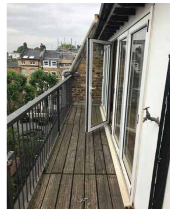
No. 178 Existing attic balcony
