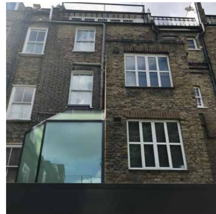
No. 178 Existing rear LGF extension
