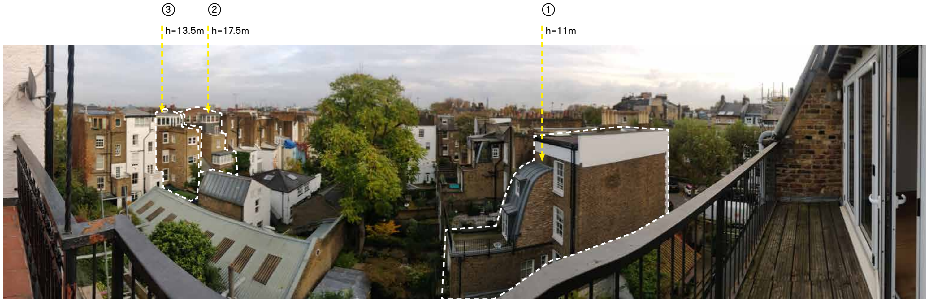
VIEW FROM SITE: THREE STOREY CLOSET WING EXTENSIONS
