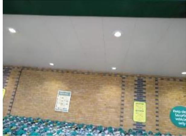
**Plate 4.9 Tightly Fitted Ceiling Tiles
