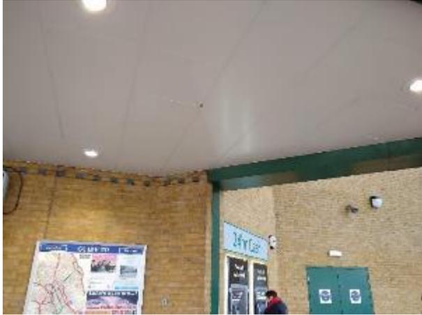
**Plate 4.8 Tightly Fitted Ceiling Tiles
