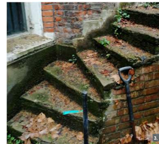
CONDITION SURVEY: 1- South Wing- Stair propped to avoid collapse. 2- North Wing- Stair supported by brickwork, cracking evident 3- Close up of damp penetration into Historic Asset
