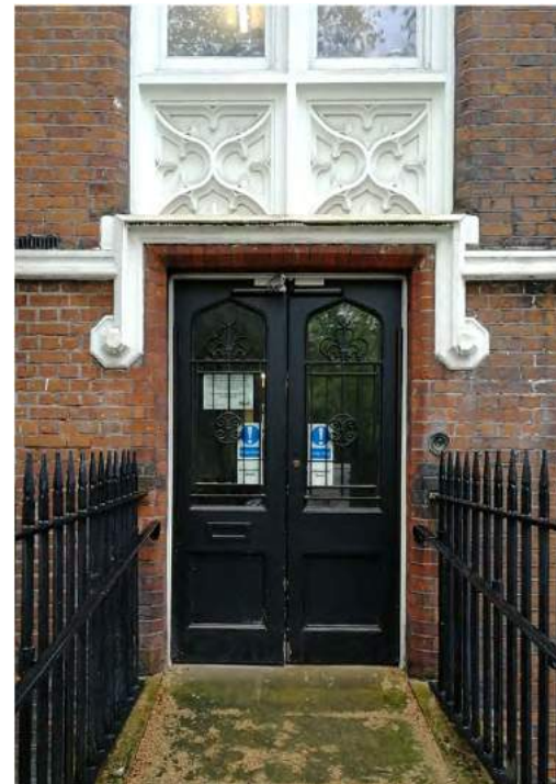
CONDITION SURVEY: Entrance door to North Wing
