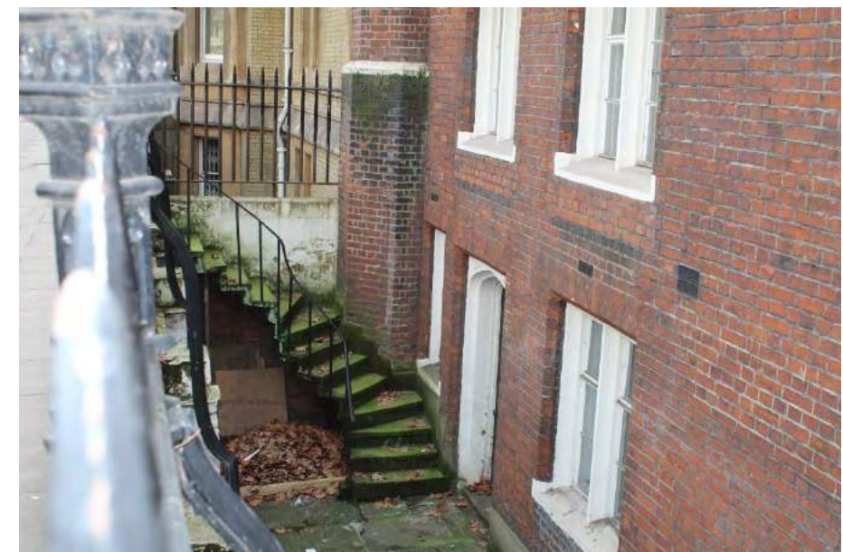
Figure 14: South external staircase
