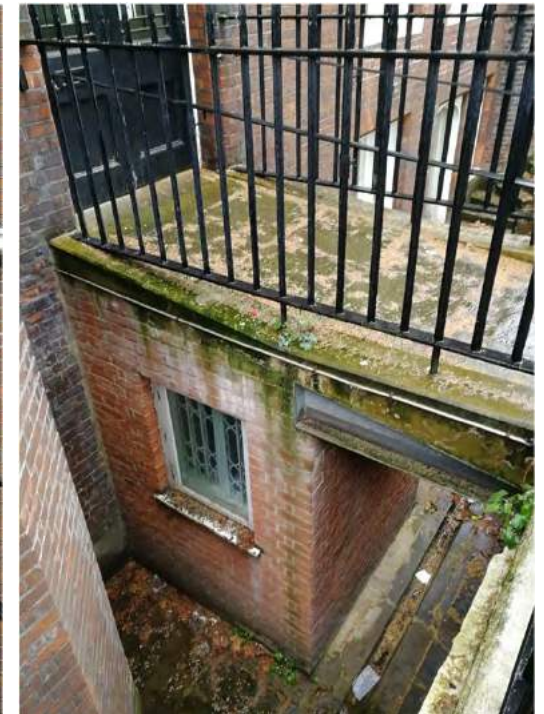
CONDITION SURVEY: North Wing Extension and Ramp
