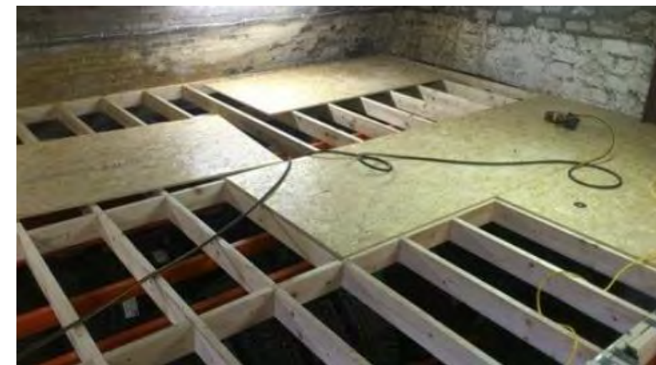
Figure 20: Example of sheathing boards placed over joists
