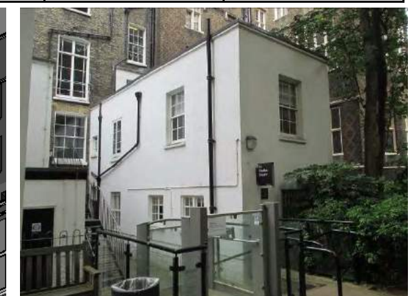
Image 9 Architects Photograph of adjacent office building
