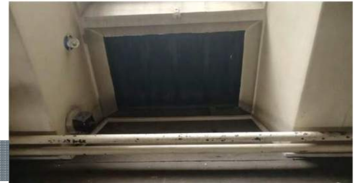
CONDITION SURVEY: Pipes running in front of window recess.
