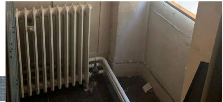
CONDITION SURVEY: Pipes running in front of window recess.
