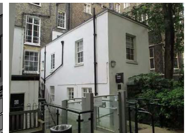
Image 9 Architects Photograph of adjacent office building
