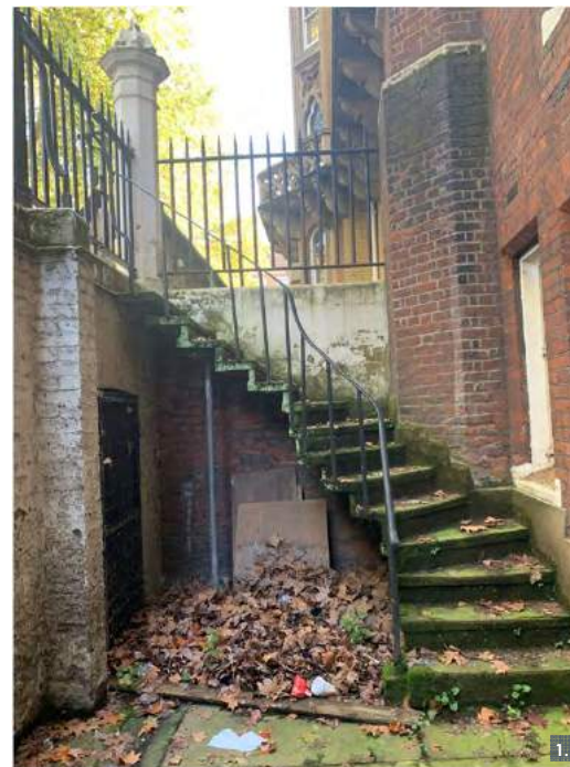
CONDITION SURVEY: 1- South Wing- Stair propped to avoid collapse. 2- North Wing- Stair supported by brickwork, cracking evident 3- Close up of damp penetration into Historic Asset
