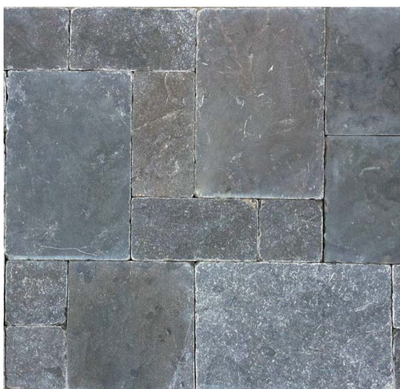
Balcony paving - Flagstones
