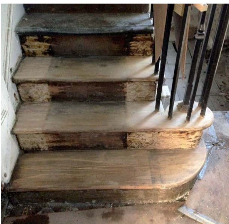
Existing Staircase - cleaned and margins repainted white, with runner added
