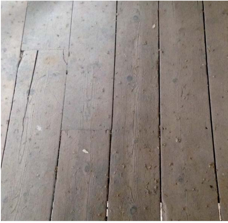
Existing Floorboard - cleaned and new finish to match engineered and bespoke board
