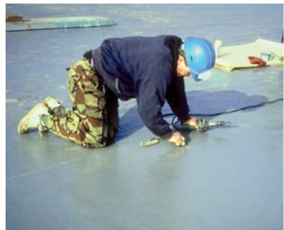
fig. 2: Verification of weld security
