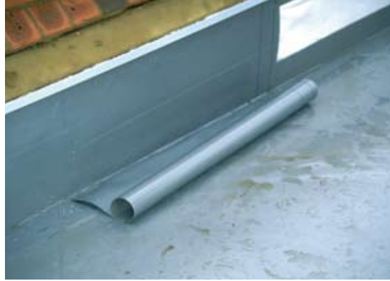
fig. 3: Edge restraint with RENOLIT ALKORPLAN 81170 or 81171 metalsheet
