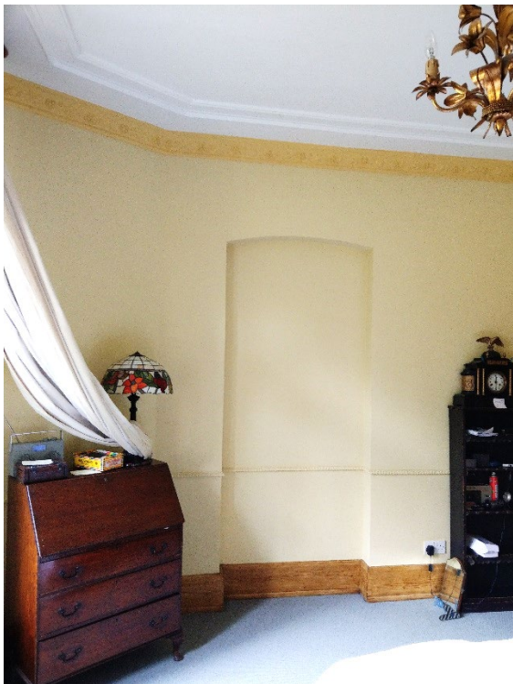
Figure 28 - Bedroom 1 - Original door, skirting and ceiling profile. Modern grape cornice.
