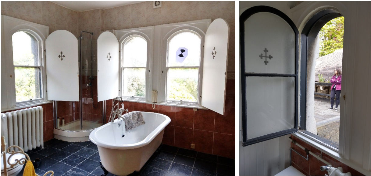
Figure 29 - Bathroom, with access to roof terrace via a window and metal bridge. Modern window shutters, finishes and ply flooring below tiles.
