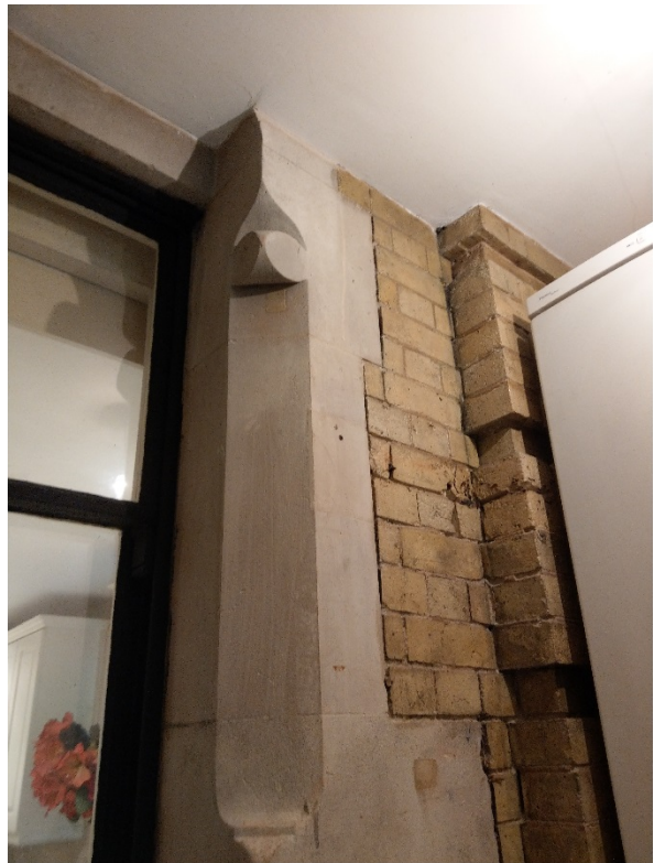
Figure 24 - Ground Floor - original window openings and external brickwork wall remain visible within 1980s porch extension, albeit modified to create a new front door during 1950s subdivision. Note the ceiling down-stand against the window in the RHS image.
