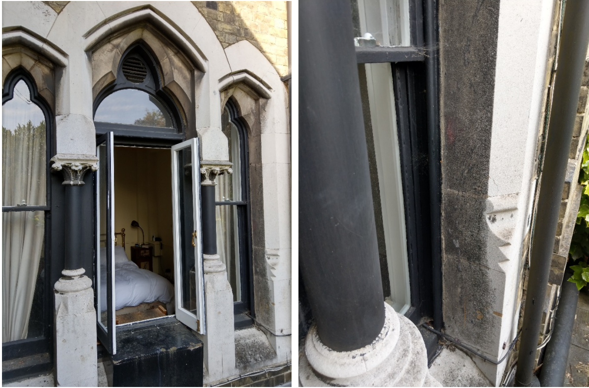
Figure 18 - Proposal - to remove unsympathetic black paint to stone and windows. Stone elements to be restored to original finish below and timber elements to be redecorated in an off-white to match immediately adjacent No.18 Well Road- providing a consistent and coherent front elevation.
