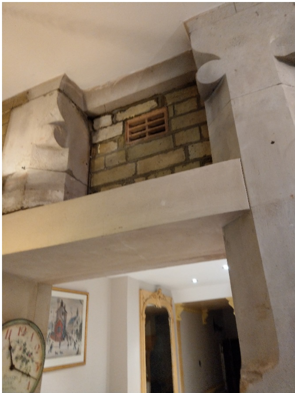
Figure 24 - Ground Floor - original window openings and external brickwork wall remain visible within 1980s porch extension, albeit modified to create a new front door during 1950s subdivision. Note the ceiling down-stand against the window in the RHS image.
