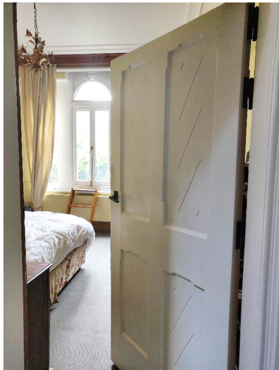
Figure 28 - Bedroom 1 - Original door, skirting and ceiling profile. Modern grape cornice.
