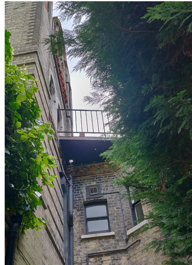
IMG 15. METAL PLATFORM - GROUND FLOOR VIEW
