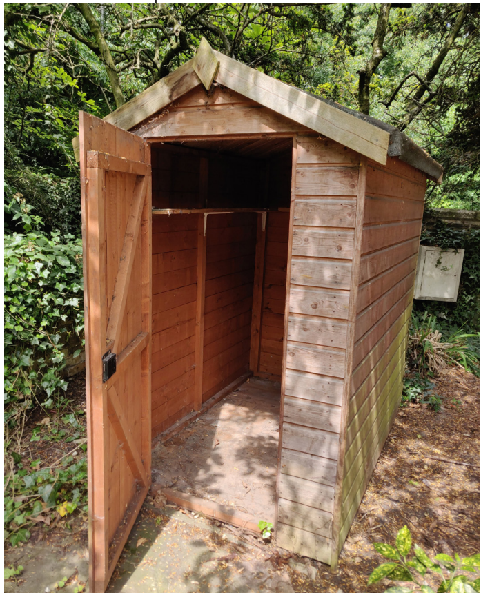
IMG 04. EXISTING SHED
