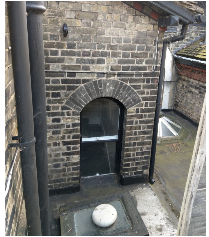
IMG 14. EXISTING STAIR WINDOW
