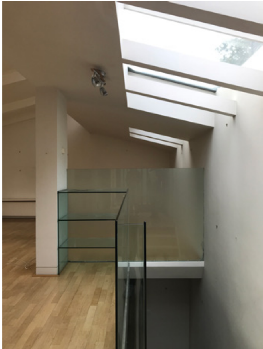
Existing rooflights over stair case
