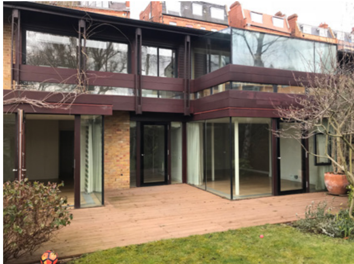
Front elevation with glazed enclosed terrace
