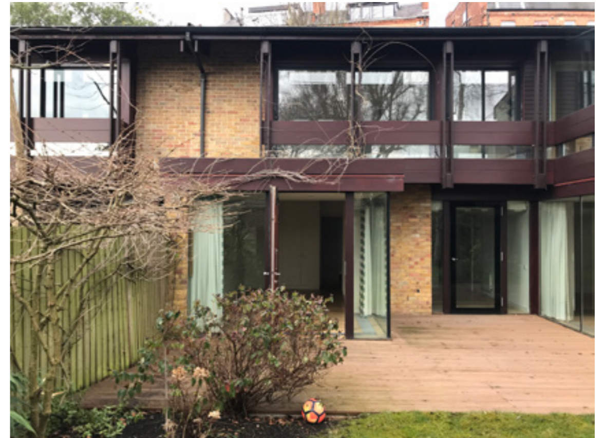
Suspended timber balcony
