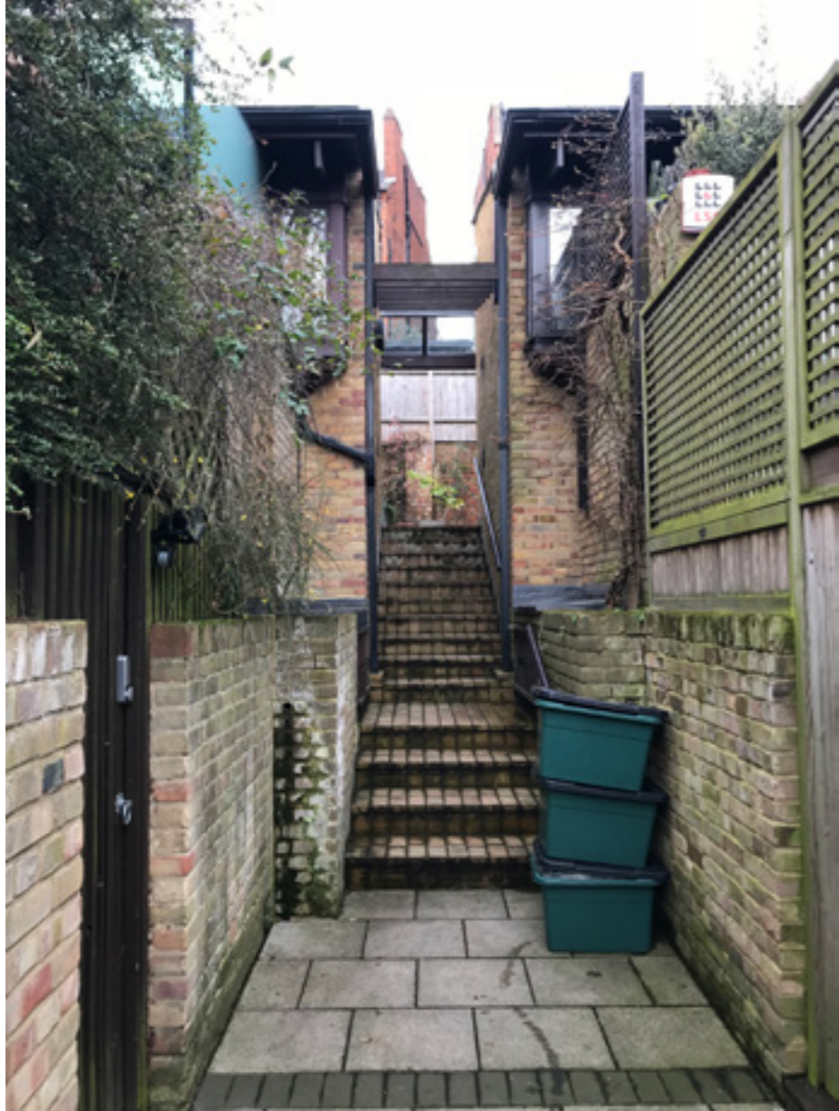
Shared passageway and steps towards entrance
