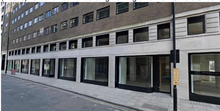
(Above): Ground floor of building fronting onto High Holborn
