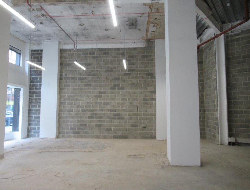
(Above): Ground floor of Unit 4B
