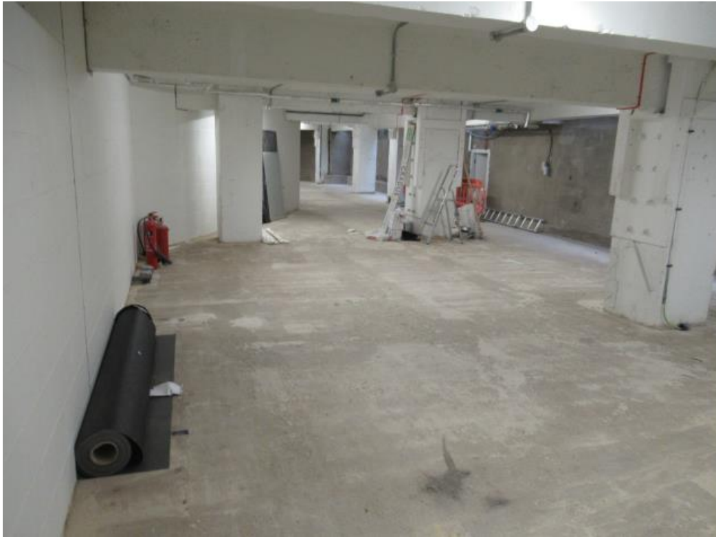
(Above): Retail storage area in Unit 4B at basement level
