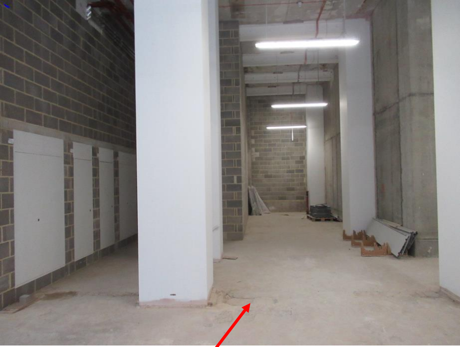
(Above): Ground floor of Unit 6
