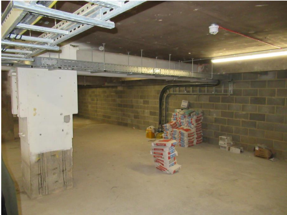
(Above): Basement of Unit 6
