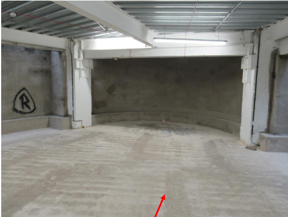
(Above): Basement area of unit 4a
