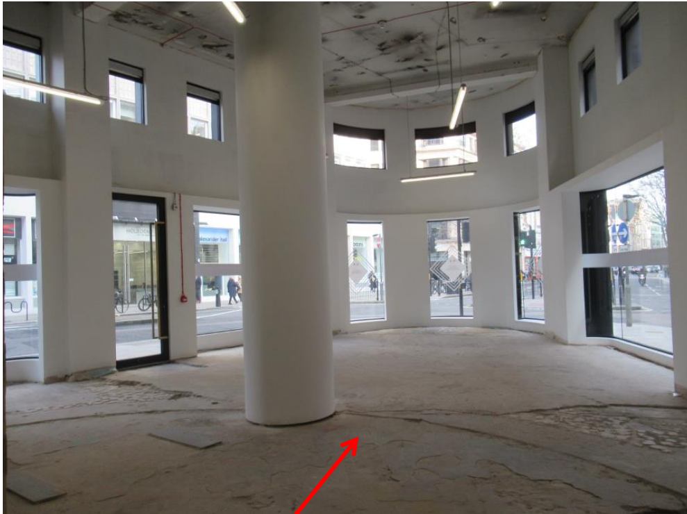
(Above): Ground floor of Unit 4a
