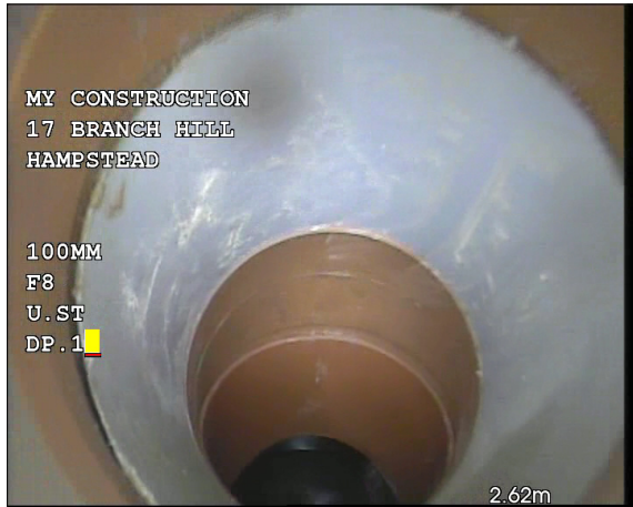
Photo: 5_5A, 00:00:01 2.62m, General observation Remarks: Floor Gully 1 Reached
