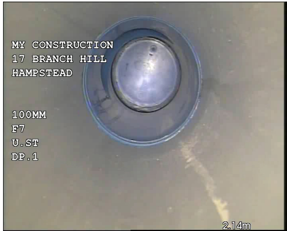
Photo: 3_6A, 00:00:01 2.14m, General observation Remarks: Drain Point 1 Reached
