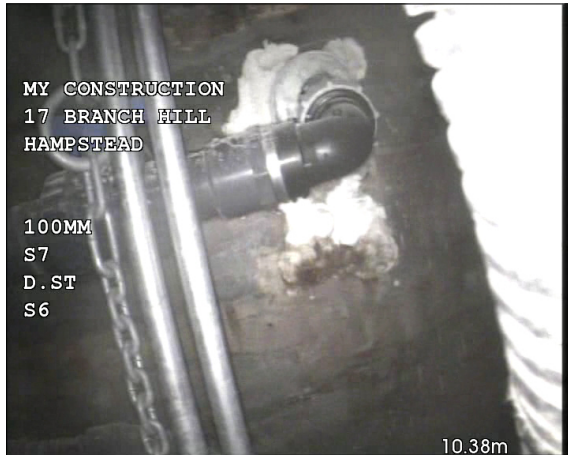
Photo: 15_6A, 00:00:01 10.38m, Manhole Remarks: S6 Reached (PS)
