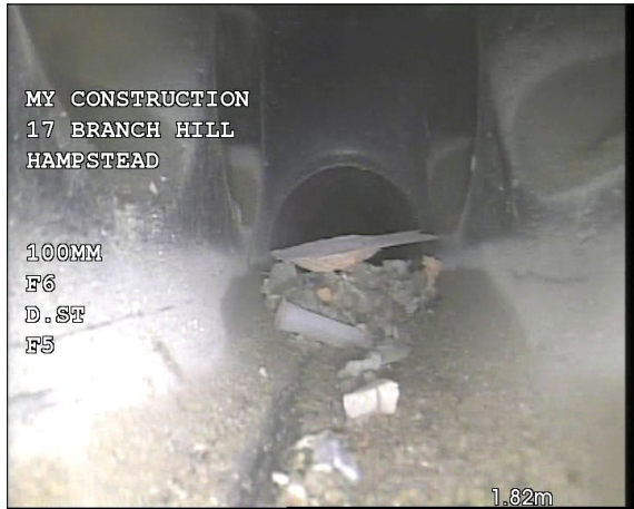
Photo: 2_4A, 00:00:01 1.99m, Manhole Remarks: F5 Reached
