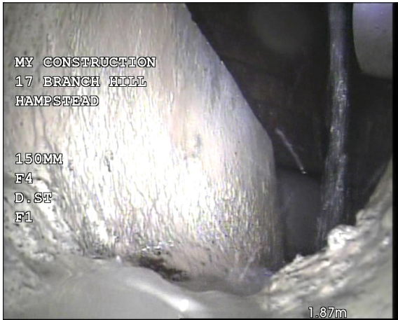
Photo: 20_4A, 00:00:01 1.87m, Manhole Remarks: F1 Reached
