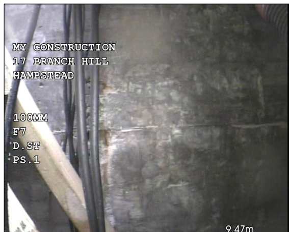
Photo: 7_4A, 00:00:01 9.47m, Manhole Remarks: PS.1 Reached
