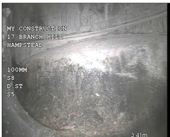
Photo: 11_6A, 00:00:01 3.41m, Manhole Remarks: S5 Reached
