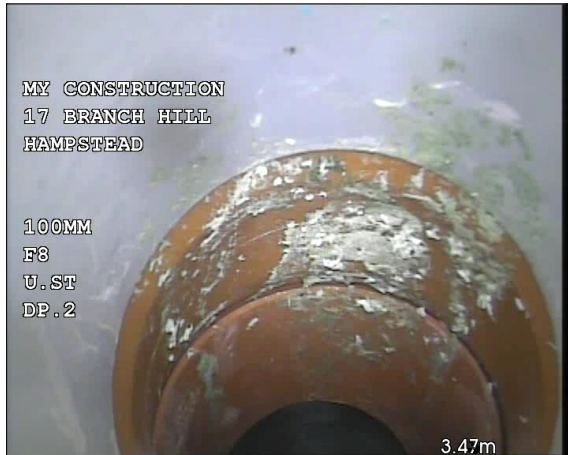
Photo: 8_7A, 00:00:01 3.47m, General observation Remarks: Floor Gully 2 Reached
