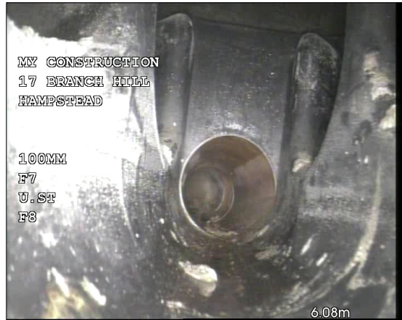
Photo: 4_8A, 00:00:01 6.08m, Manhole Remarks: F8 Reached
