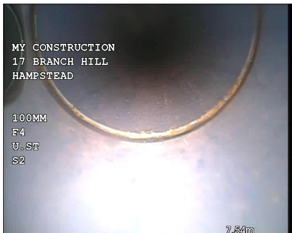
Photo: 17_6A, 00:00:01 7.54m, Manhole Remarks: S2 Reached
