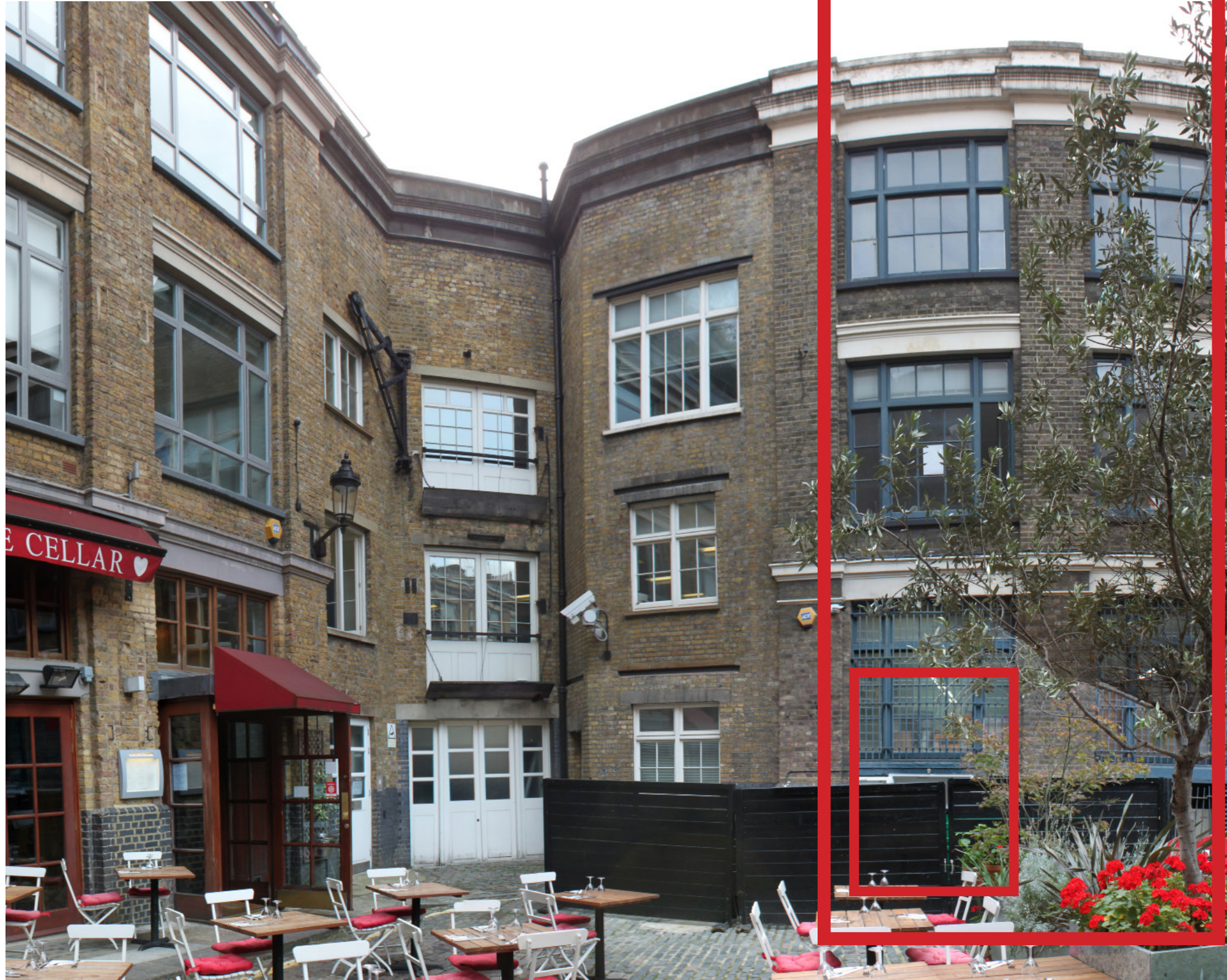
5 Bleeding Heat Yard
