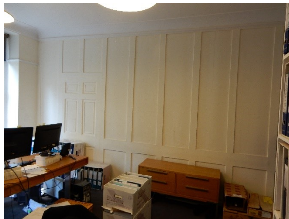
North Wall of Room F3/F4
