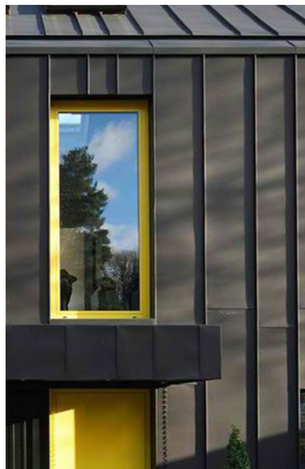
Fig.8 - An example of the type of dark metal standing seam cladding proposed to the walls and roof of the extension.
