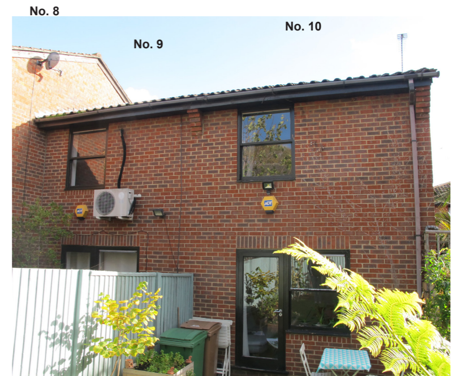
Fig.4 - photograph of the rear of the terrace as viewed from the garden
