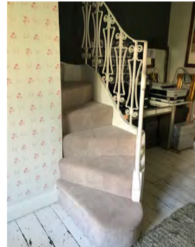
2. Existing stair to first floor - its footprint it believed to have altered from the original and the banister has been replaced.
