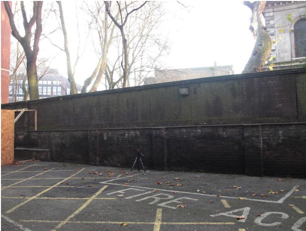
Wall from Car Park Side 45 New Compton Street
