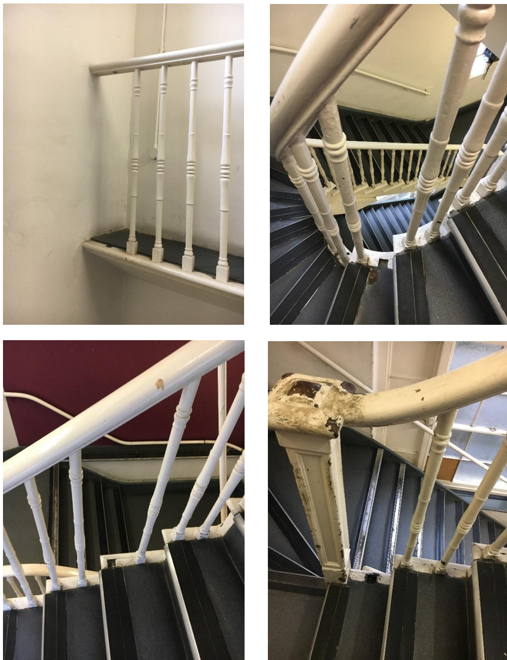
Figure 5.2: Missing Spindles to be replaced at third floor level (top) and first floor level (bottom) exact location detailed in Figure 5.1
