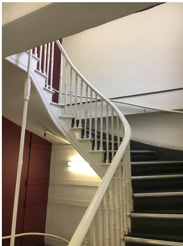
Figure 3.8: Staircase within Block C leading to third floor level, missing spandrel towards the top
