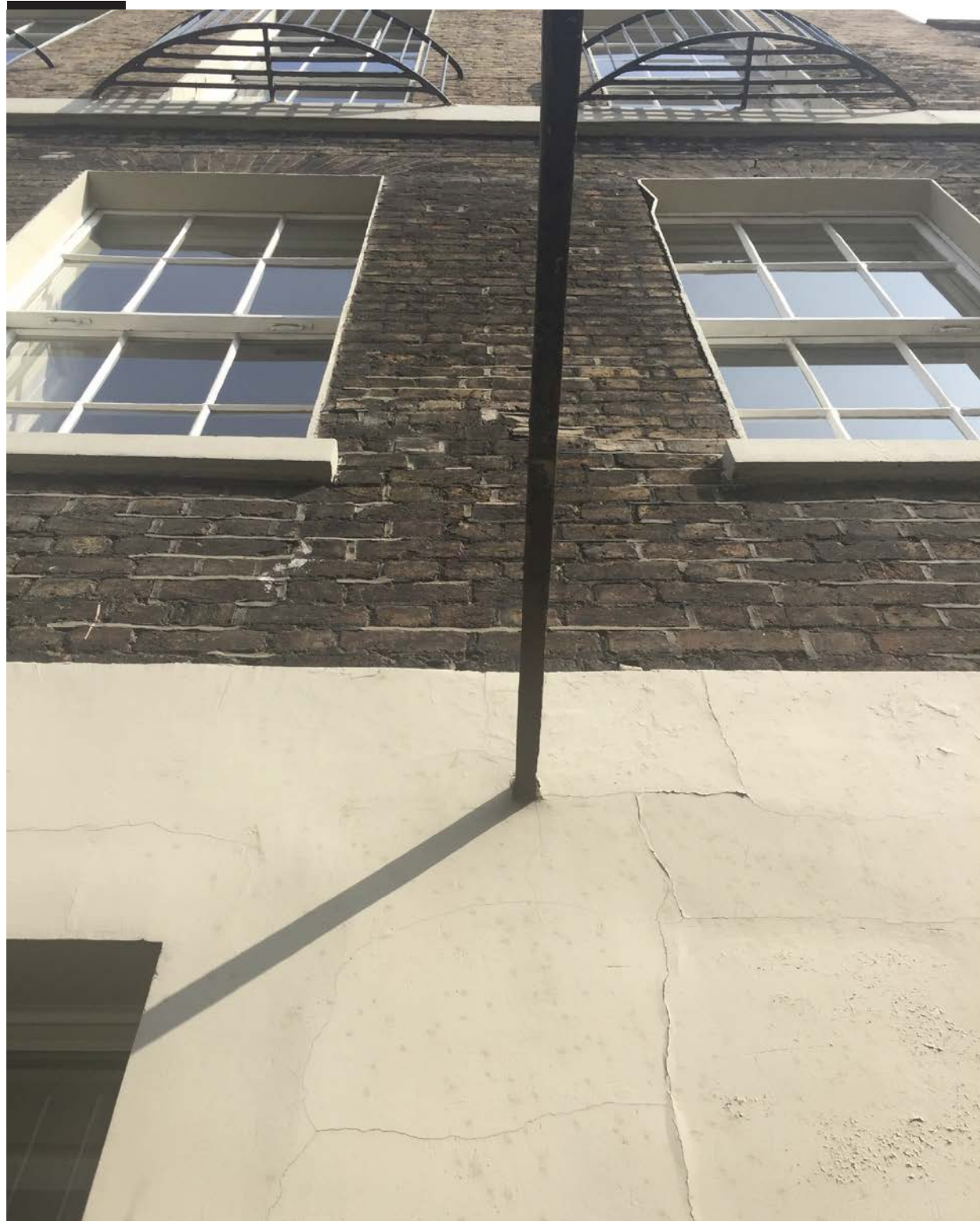
Existing modern sand/cement render on Conway St elevation (before demolition)
