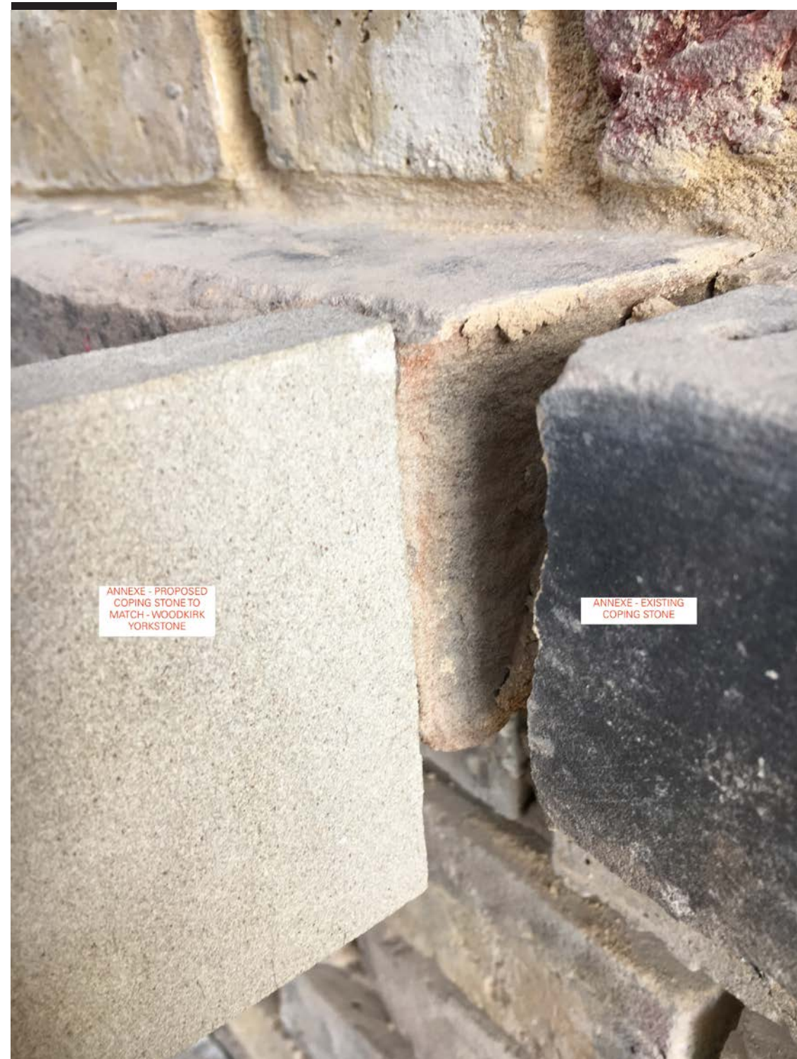
Existing Yorkstone coping and proposed replacement Yorkstone for sills & coping
