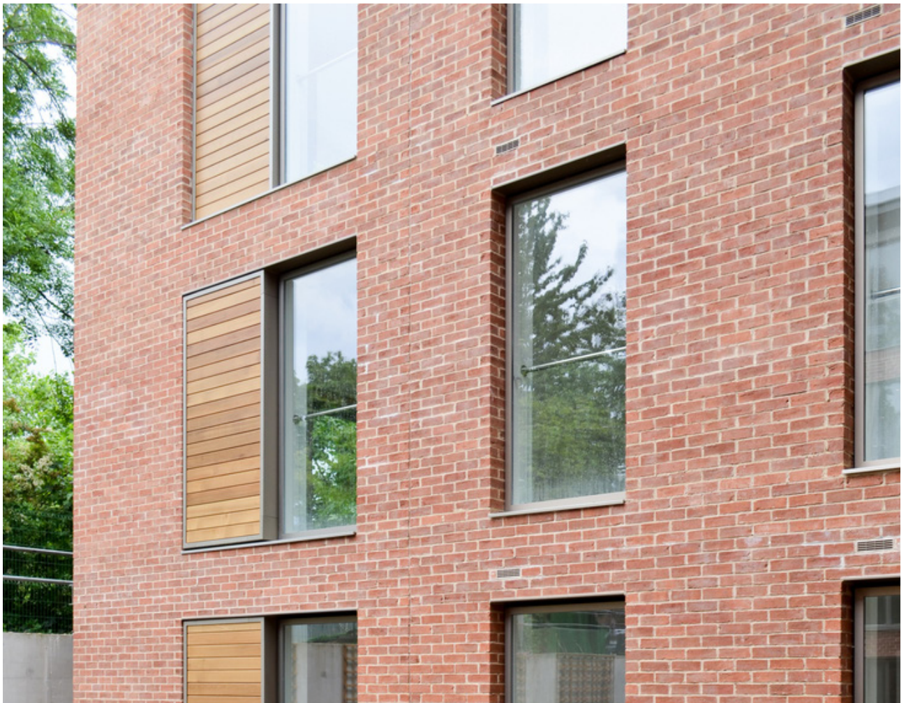
Western Red Cedar boarded infill panels to window frames in Beaufort House
