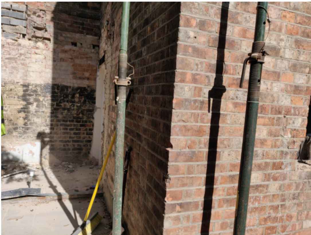
Photo 2: Rear of existing outrigger
