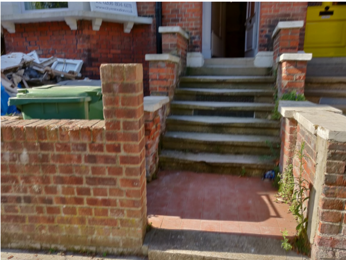
Photo 4: Stairs to be repaved
