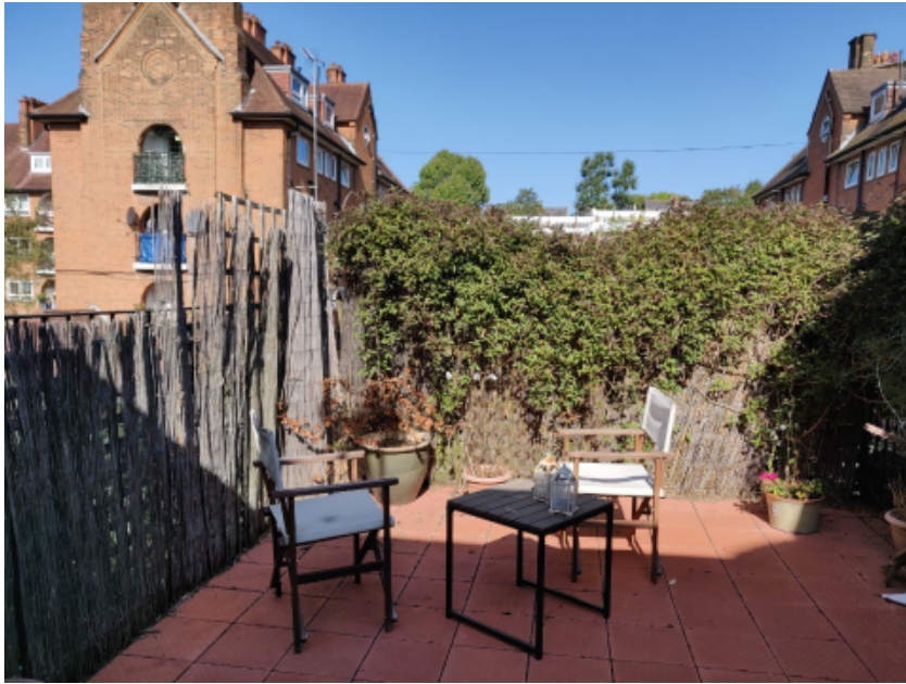
Photo 3: Existing rear terrace
