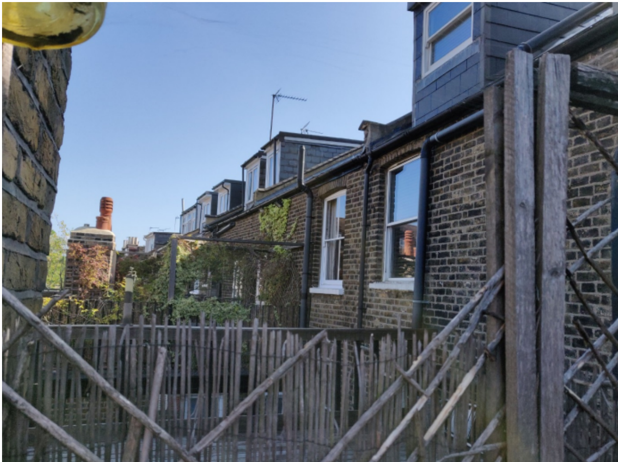
Photo 4: View of dormers looking eastwards from the terrace
