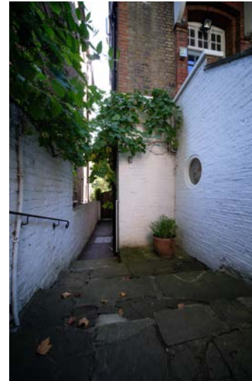
VIEW TOWARDS SIDE PASSAGEWAY
