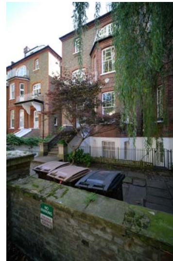
STREET VIEW TOWARDS FRONT LIGHTWELL
