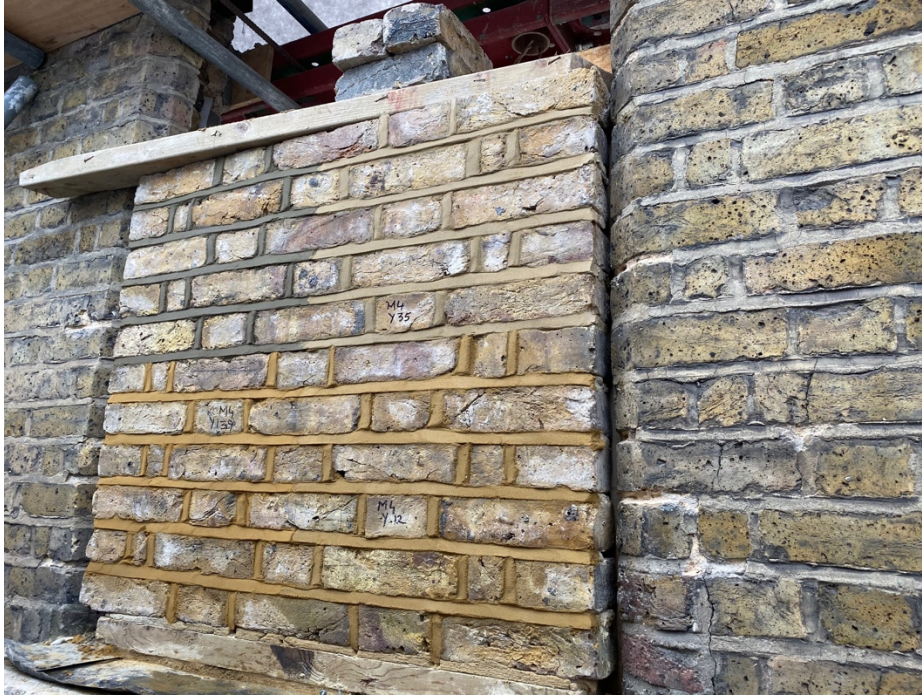
Sample brickwork panel using original bricks built between existing/retained facade showing four samples of pointing - proposed choice of pointing is labelled 'M4 Y35'
