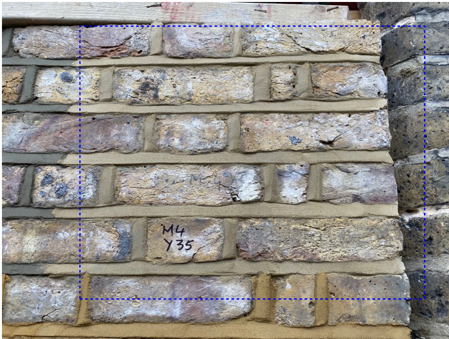
Pointing to existing/retained facade is not original, varying in colours / textures and is in poor condition. The proposal is to repoint the entire facade with the selected pointing so that all matches.
