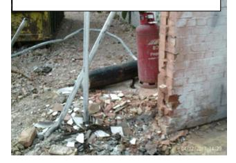
The demolition arising currently on site will be stockpiled by means of a 360 degree excavator and placed away from the site operations ensuring that all access routes are clear of debris and level so far as is reasonably practicable.
