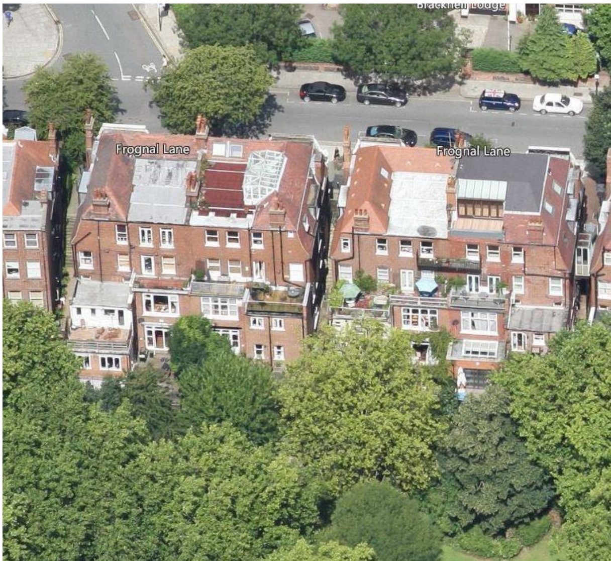
Fig.4 - Birds eye view illustrating roof level development at no. 12 and no. 16 Frognal Lane.
