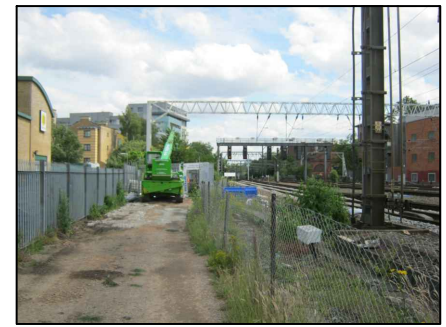
PHOTO 1 - VIEW FROM HIGH MILEAGE APPROACH ACCESS TRACK TOWARDS THE VAULTS
