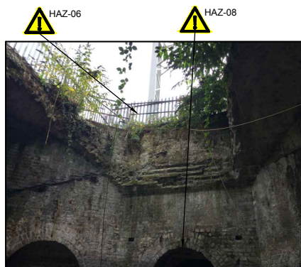
PHOTO 5 - VIEW FROM EAST BOILER ROOM UP THROUGH COLLAPSED ARCH
