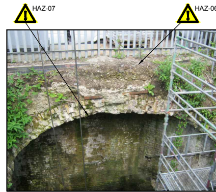
PHOTO 4 - VIEW INTO EAST BOILER ROOM THROUGH COLLAPSED ARCH
