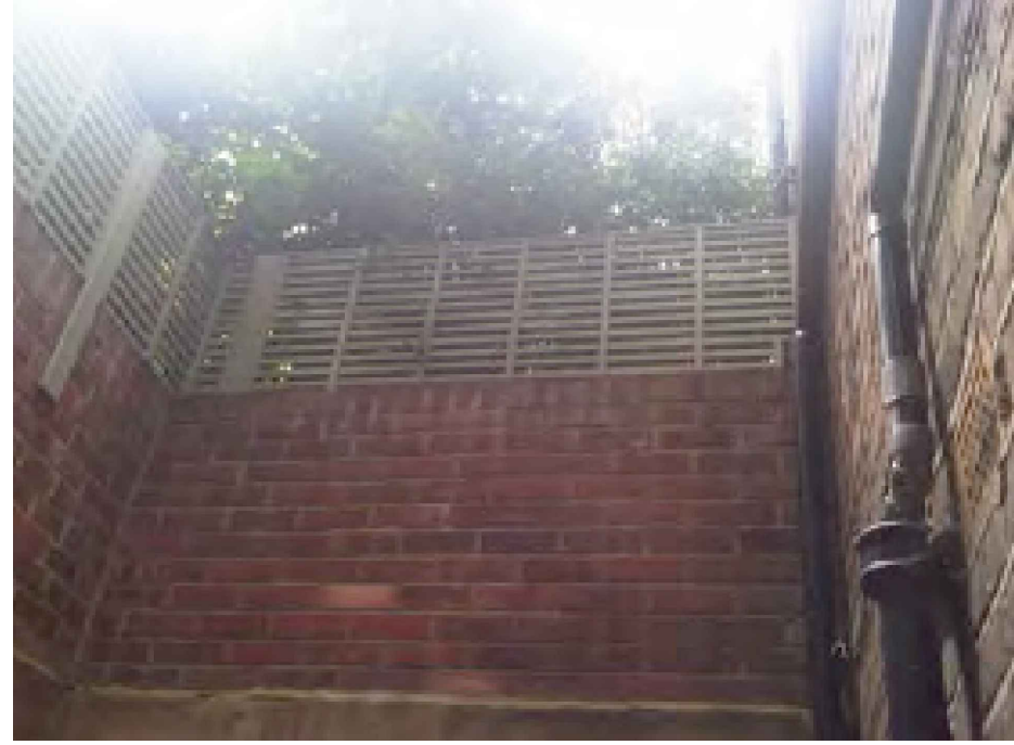
IMAGE OF EXISTING LIGHTWELL LOOKING TOWARDS TENANTS ABOVE FENCED TERRACE
