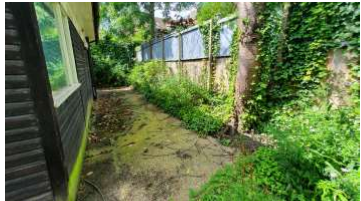
Showing base of T5 & T6 adjacent the outbuilding
