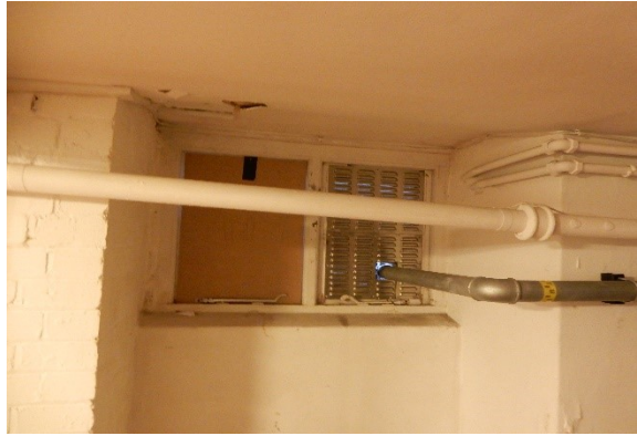
Modern timber casement windows
