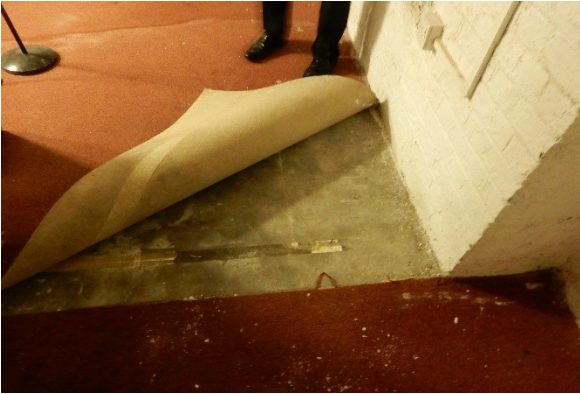
Modern concrete slab below carpet
