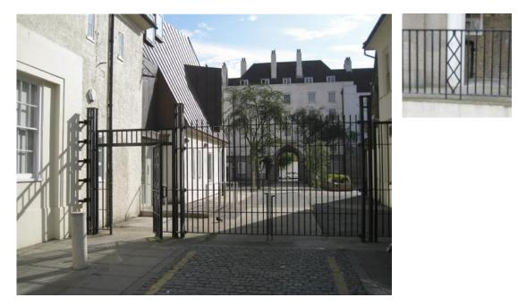
The proposed gates and railings will be completely reversible so could be removed at some future date without detriment to the original fabric or design.
