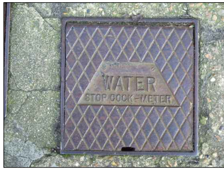
FIG 5 - STOPCOCK AND WATER METER COVER
