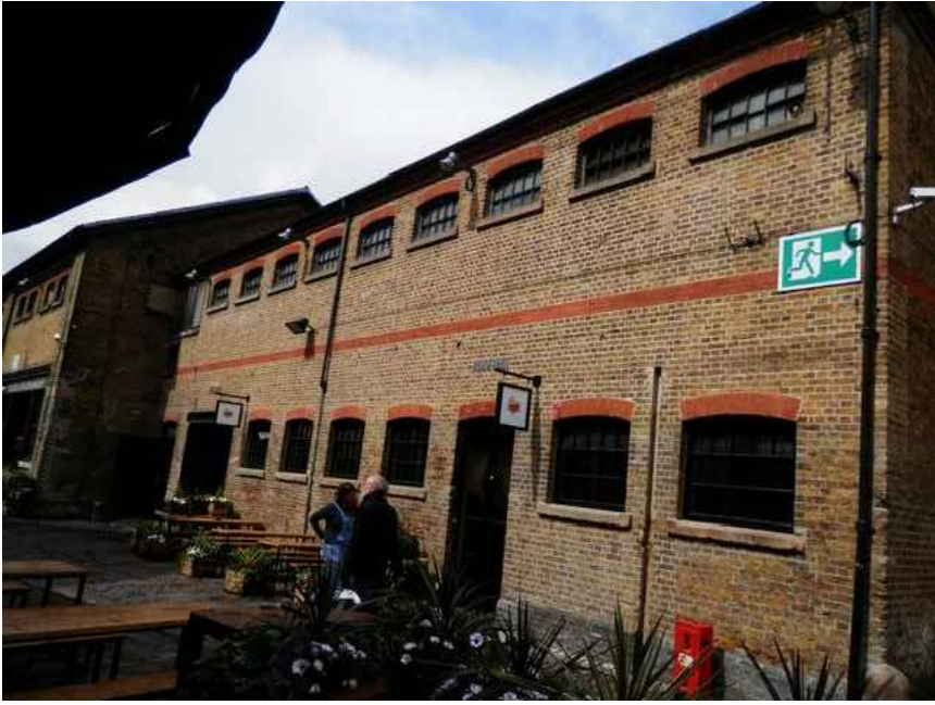
FIG 7 - EXISTING H/L IGUZZUNI LUMINAIRES TO BE RETAINED. EXISTING EXTERNAL LIGHTING CABLING TO BE REMOVED AND REROUTED INTERNALLY WITHIN THE BUILDING. LOW LEVEL FLOOD LIGHT TO BE REMOVED
