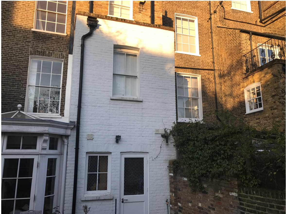
View of rear elevation bay to be underpinned
