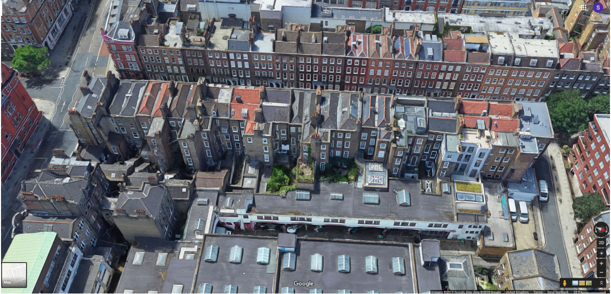
Fig.05: Existing building: 14 & 15 Great James St, highlighting the rear closet storeys
