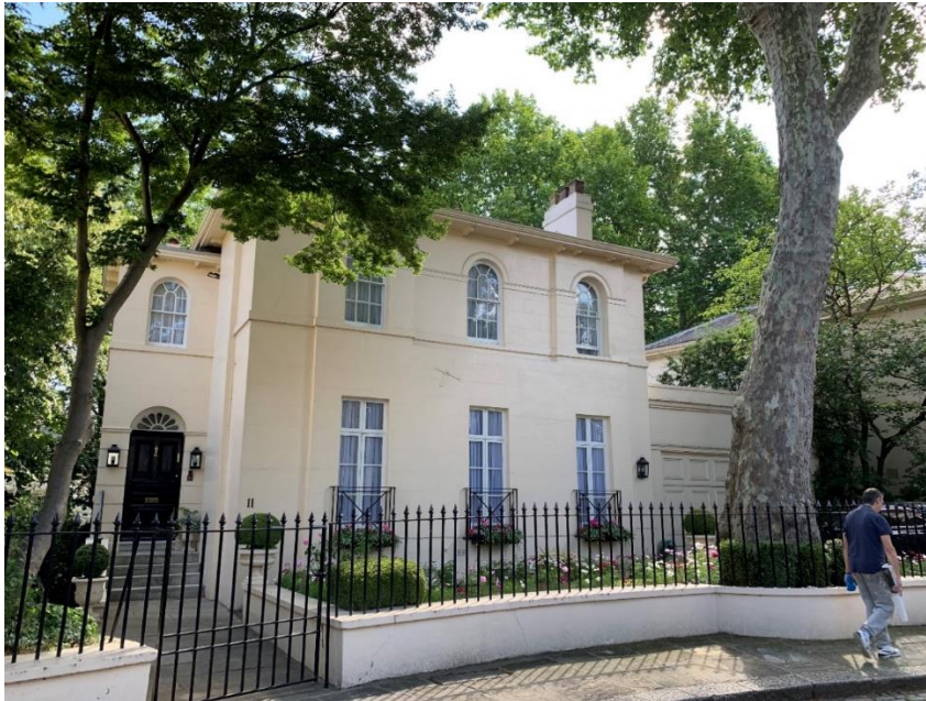
Figure 1- View of the property from Park Village West
