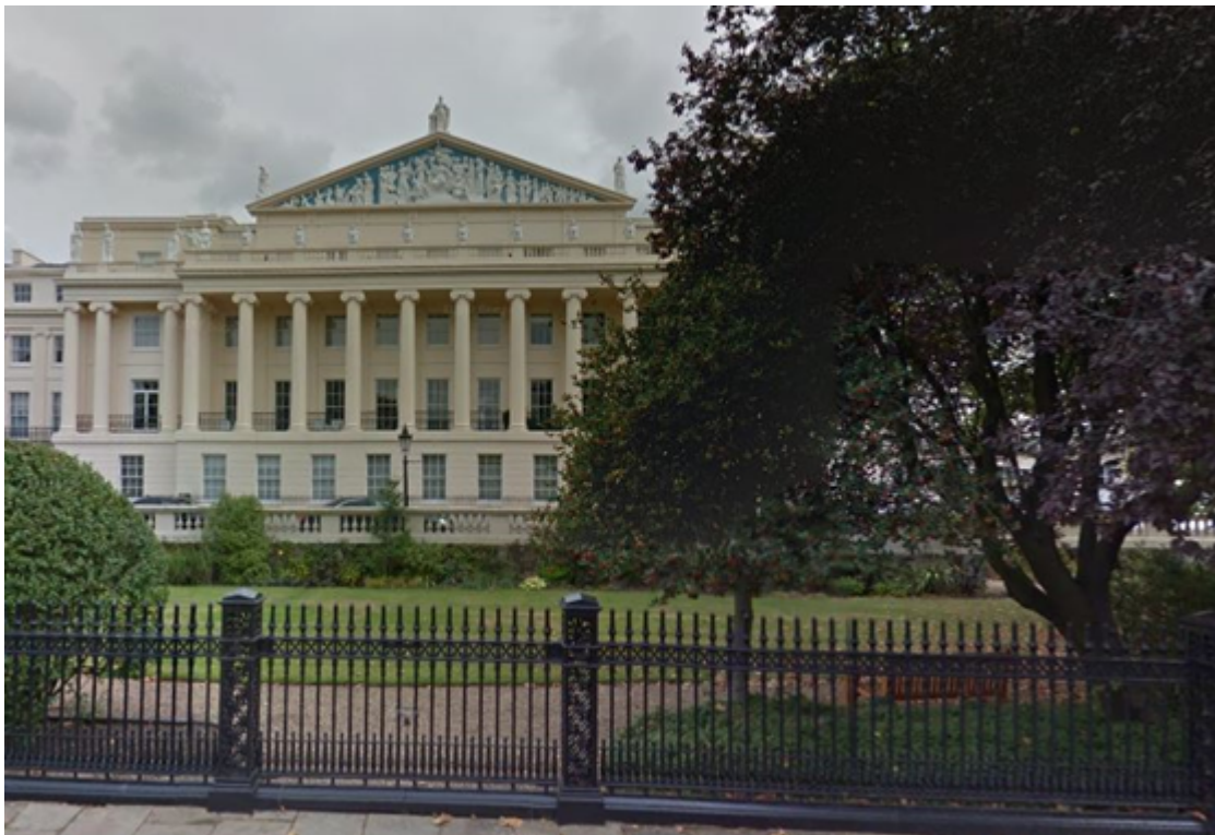
Figure 1: site photo from the Outer Circle.
