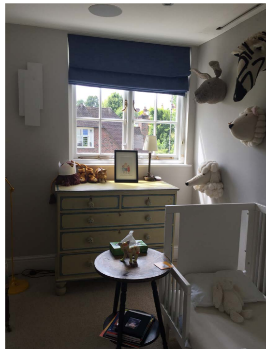
2.&3. Existing partition wall to be reinstated to original position and gable window adapted to accommodate.
