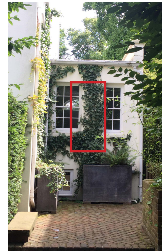
Existing Entrance Porch - Rear Facade
