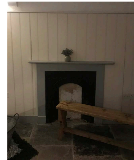
13. Keats House bead & butt lower ground floor wall details to be used as precedent.
