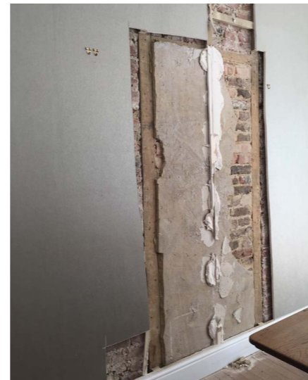
14. Opening-up works reveal original doorway between front rooms - to be reinstated.
