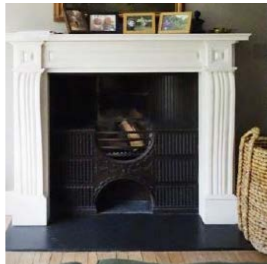
13. Modern fireplace - to be replaced (original grate to be retained)
