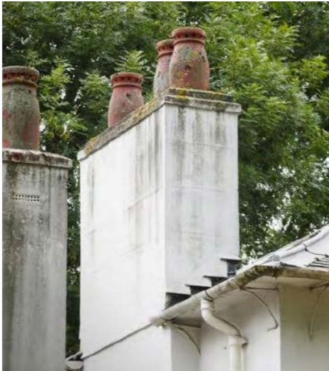
Keats House scored stucco, chimney pots & original rainwater goods
