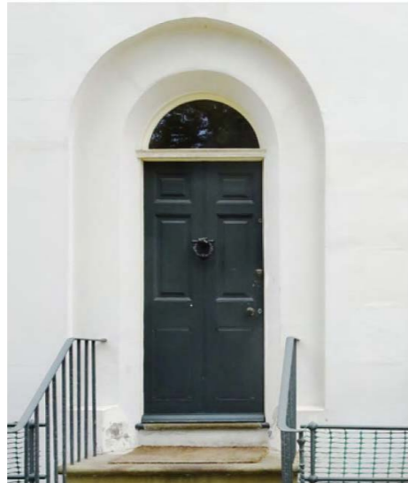
Keats House main entrance front door - precedent for new entrance door panelling
