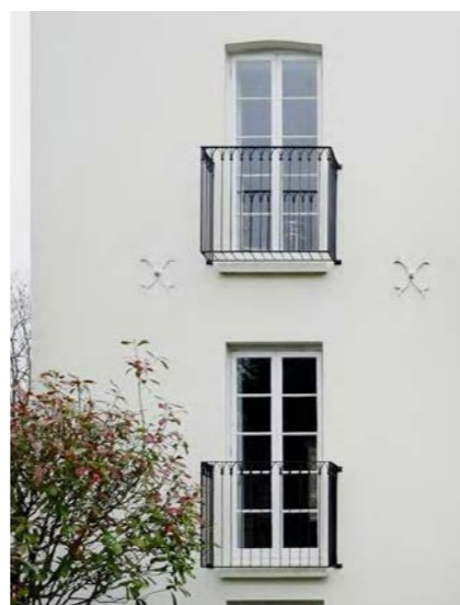
5.2.6 Existing modern rear balconies
