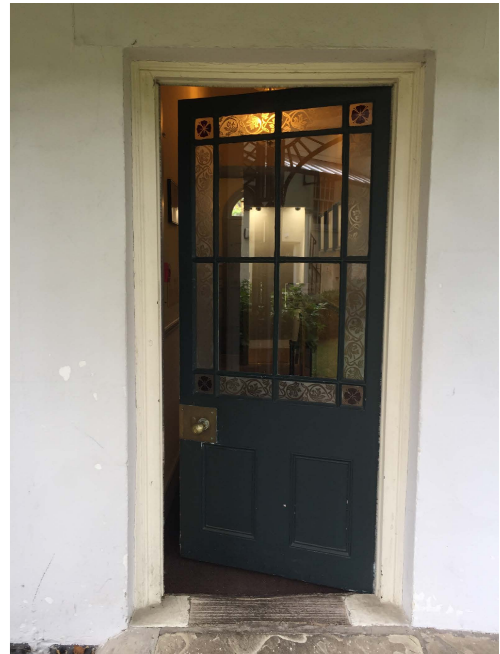
Keats House Garden Door - external view
