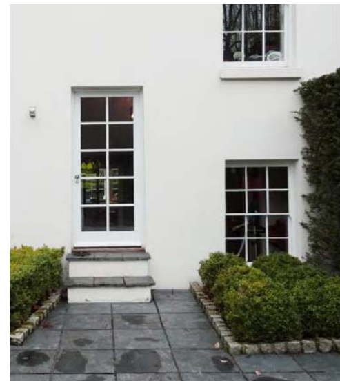
5.2.5 Existing modern rear garden door
