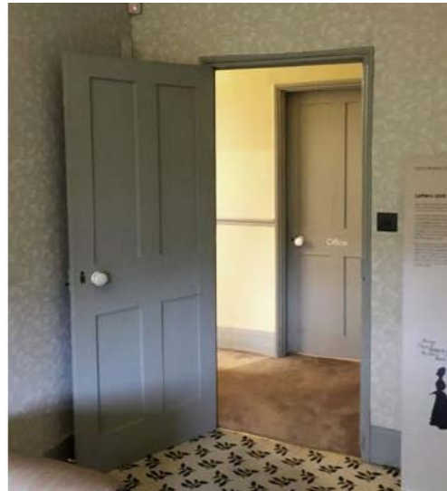
Keats House first floor doorway detailing
