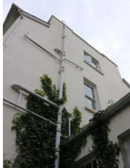
5.2.4 Existing plastic rainwater goods & pipes
