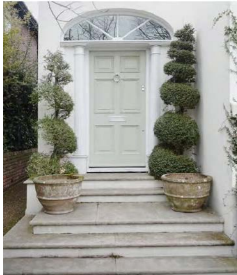
5.2.1 Existing modern front door & fanlight
