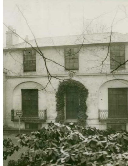
5.2.8 Keats House with dark window frames
