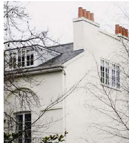
5.2.2 Existing synthetic smooth stucco & modern chimney pots
