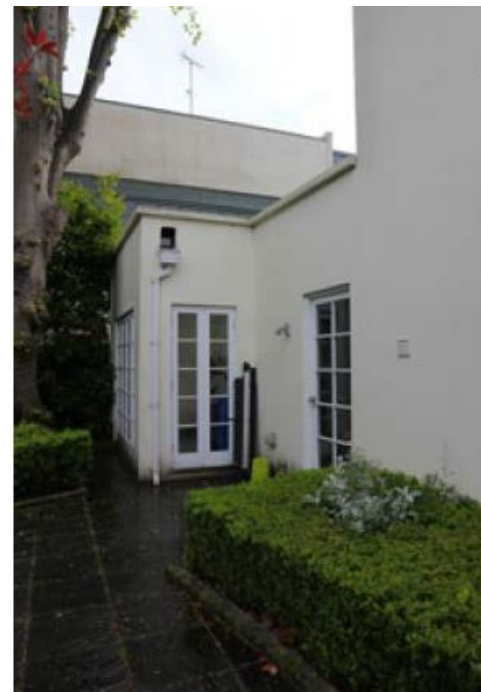
3. View towards eastern garage extension
