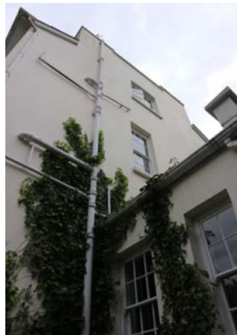
1. West Facade - showing greenery & pvc downpipes
