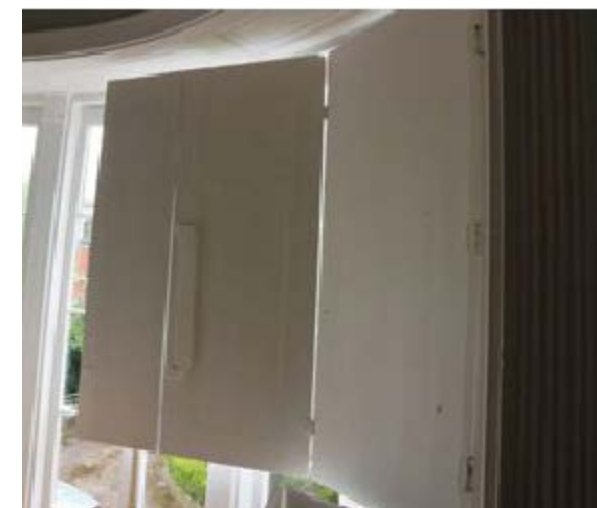
3. Drawing Room - original timber window shutters on elliptical bay
