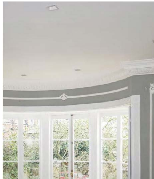
Modern plasterwork and downlights
