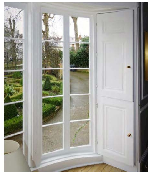
Modern windows with chunky frames, next to original shutters
