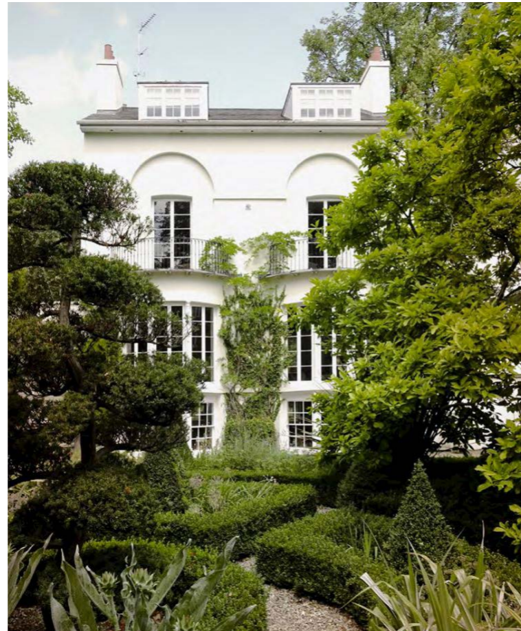
2. Front Facade - viewed through formal front garden planting
