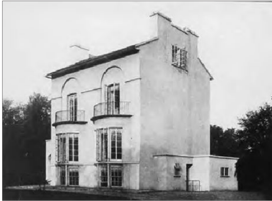
Front and East Side Facades, 1920
