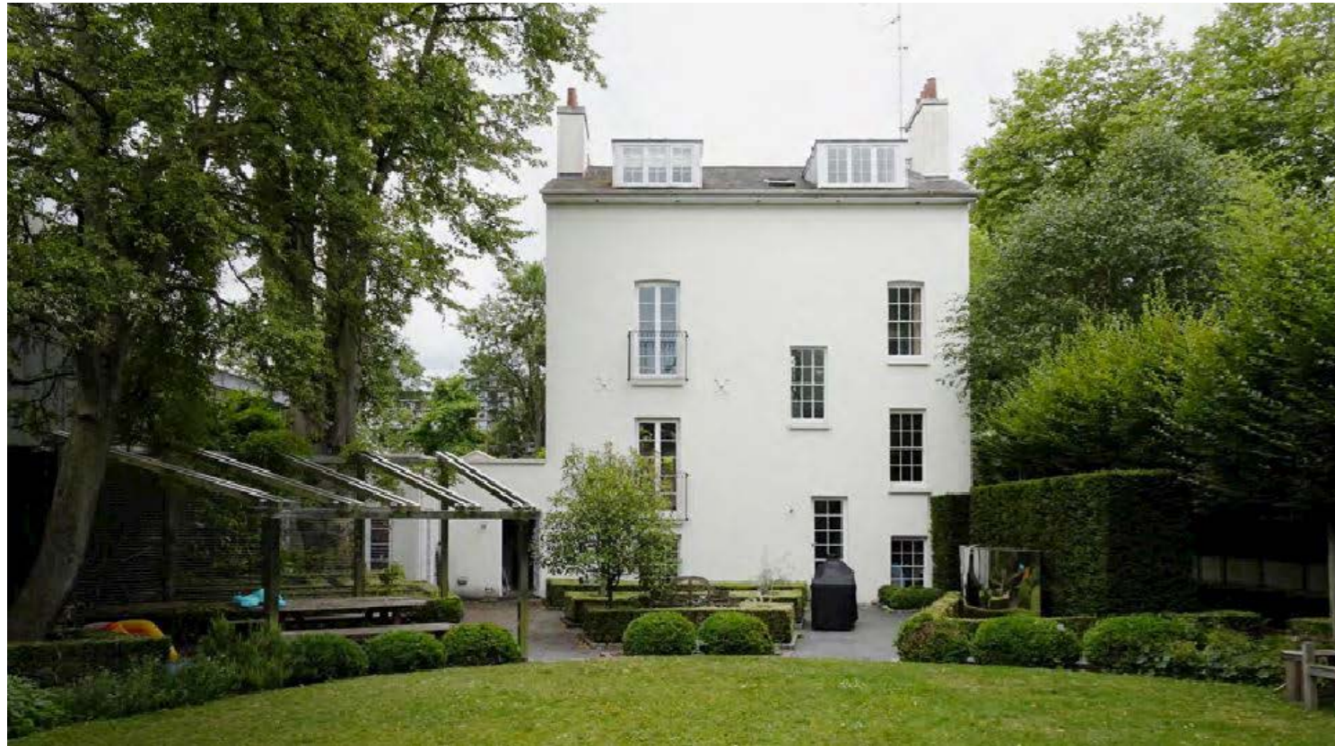
1. Rear Facade - viewed from rear garden
