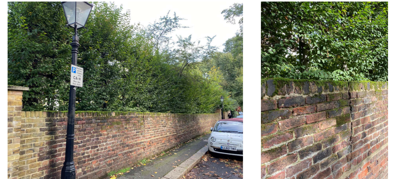
No.12 Keats Grove - View from Keats Grove pavement - highlighting the brick garden wall and natural privacy screening provided by the front boundary planting. The wall is most likely original but has been substantially modified by extensions; as evident by a change in course, infills, and repairs.
