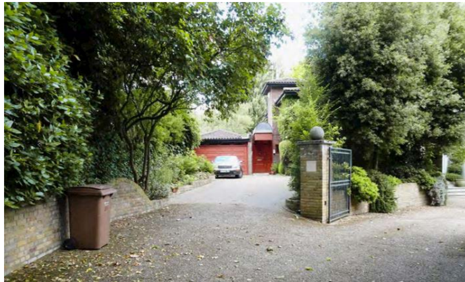
No.12B Keats Grove - Front view from shared entrance driveway
