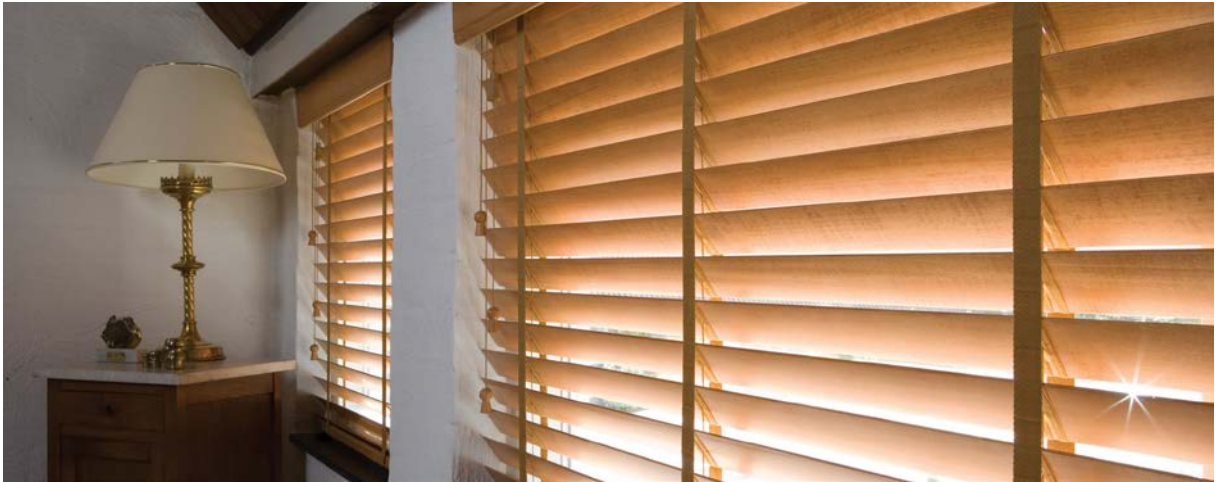
Figure 3: Example of venetian blinds angled downwards to reduce solar gain
